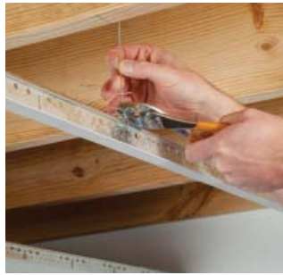
2 Suspend main beams with hanger wire
