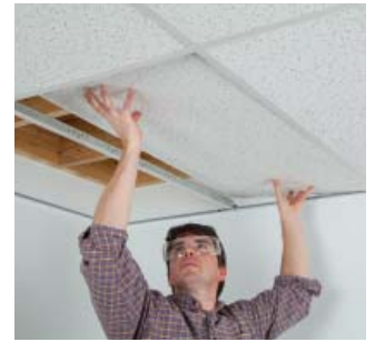
4 Install ceiling panels
