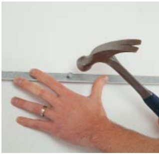
1 Install wall moldings
