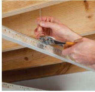
2 Suspend main beams with hanger wire
