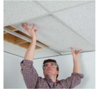
4 Install ceiling panels
