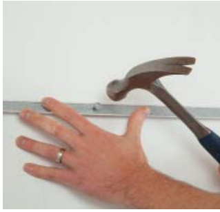
1 Install wall moldings
