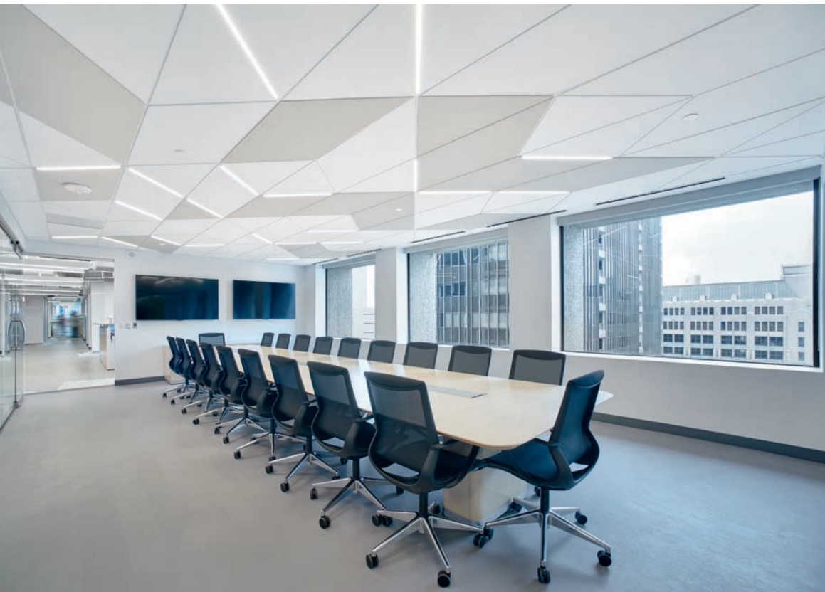
▲ Calla® Shapes panels with Suprafine® XM 9/16" suspension system
