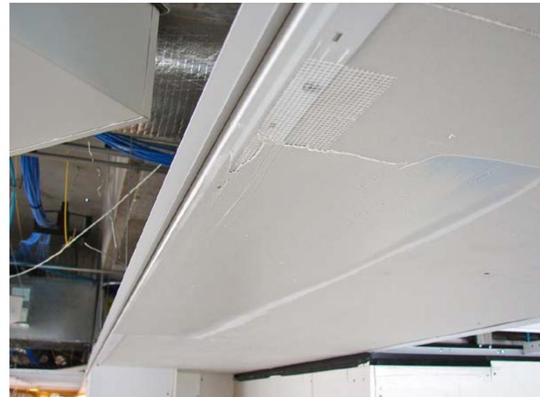
*As with our Steel Transitions, mesh or paper tape can be used to ensure cracking doesn't occur.*
