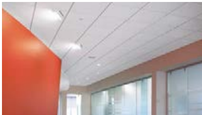
Flat, level ceiling with standard acoustical suspension
