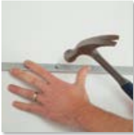
1 Install wall moldings
