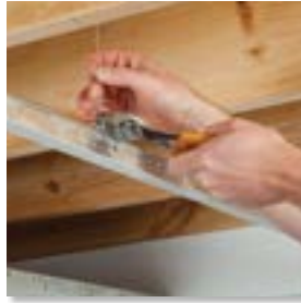
2 Suspend main beams with hanging hardware
