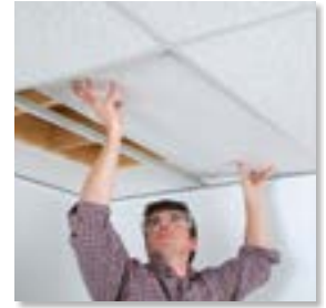
4 Install ceiling panels
