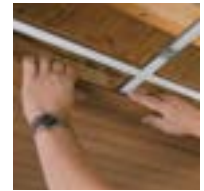
Position planks; slide and secure clips
