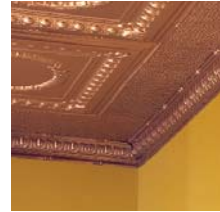
FILLER PANEL AND CORNICE APPLICATION
