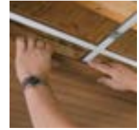
Position planks; slide and secure clips
