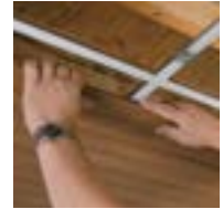
Position planks; slide and secure clips
