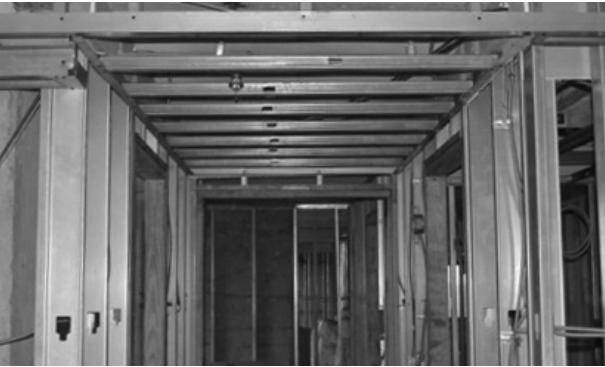
Corridor framing using traditional steel studs
