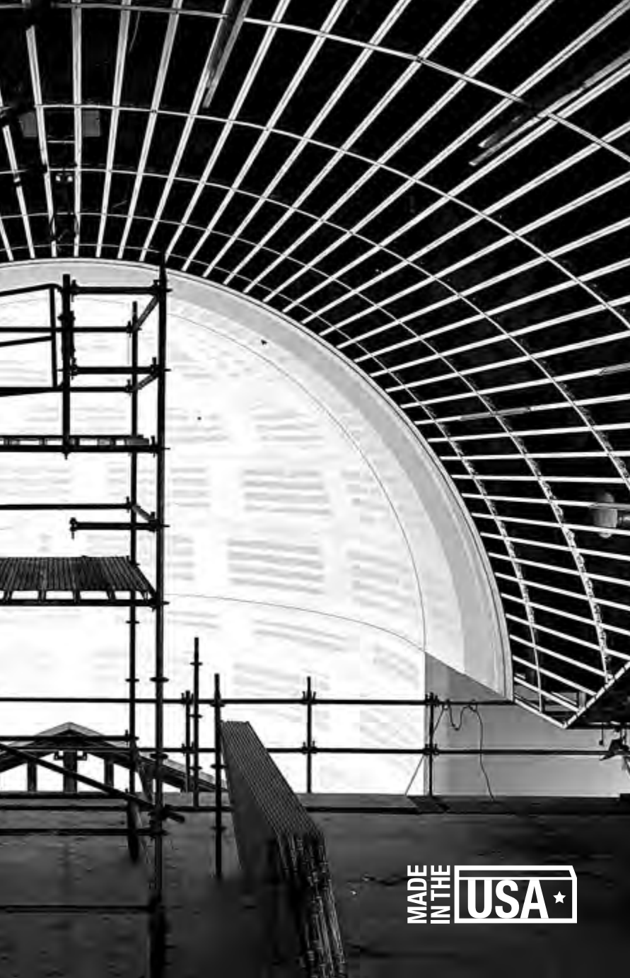
Flat Drywall Grid barrel vault installation
