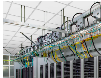
DynaMax Structural Aluminum Data Center Suspension System
