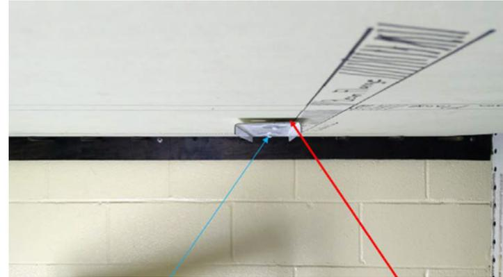
(Fig 3) Temporary Retaining Bracket installed
