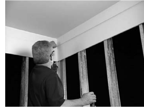
Mark desired height for new ceiling
