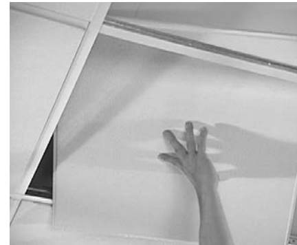
Tilt panels above frame and drop into place
