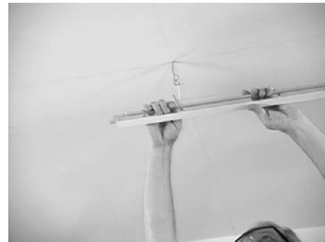
Install first main beam
