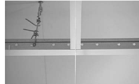
Align second guide string with first four-foot cross tee
