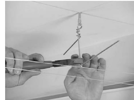
Bend hanger wires at height of guide string
