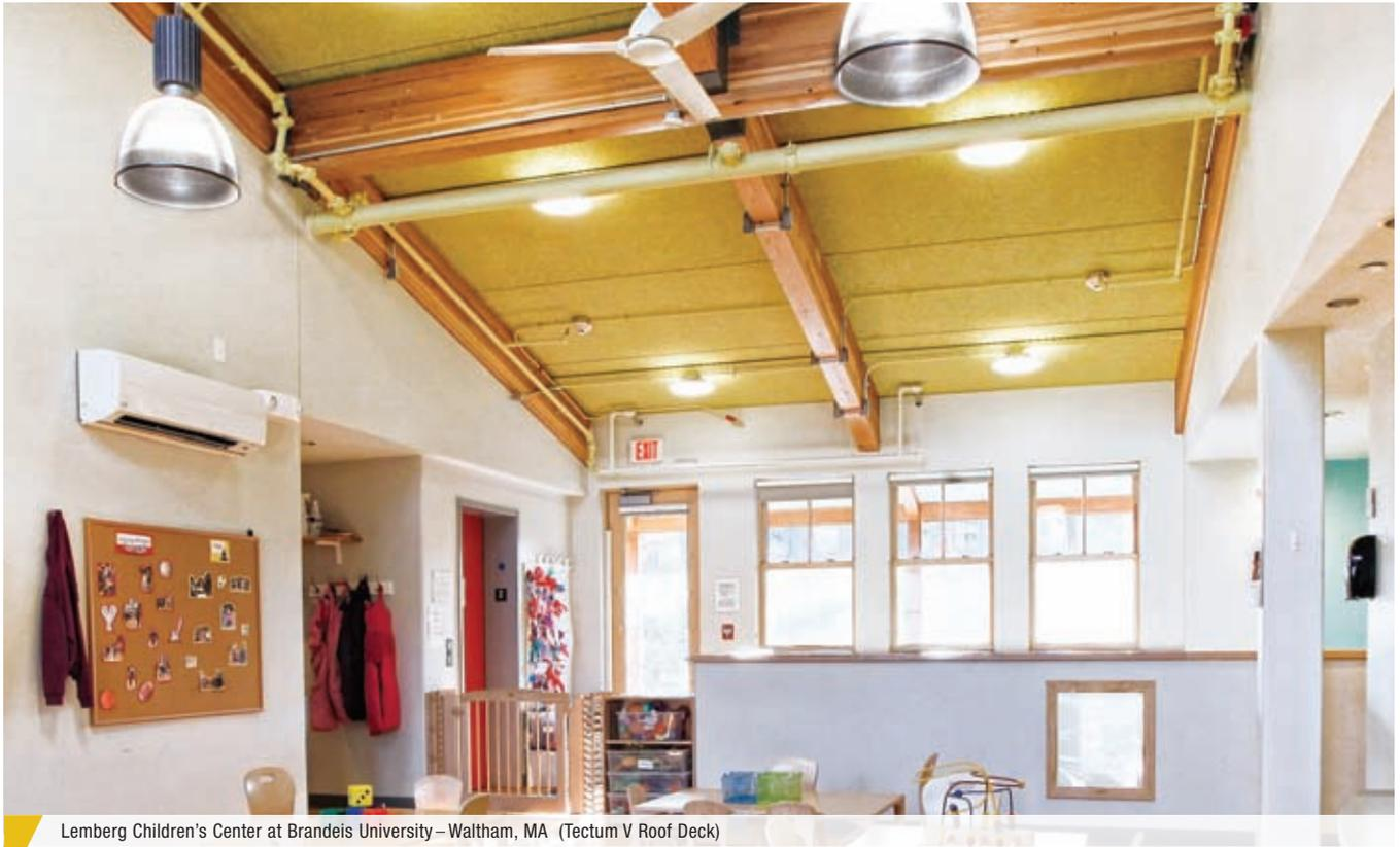
Three-in-One Composite Roof Deck Panels provide acoustics, insulation, and a nailable surface that accepts a wide variety of roofing materials.
