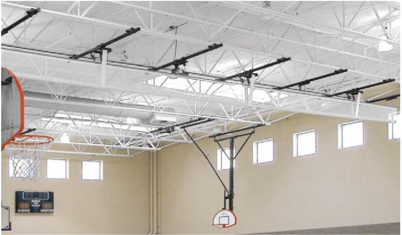
East Lawrence Recreation Center – Lawrence, KS (Tectum I Roof Deck)
