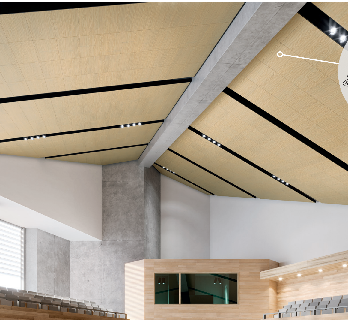
MetalWorks™ Airtite® Radiant AR-B 2' × 4' panels in Effects Ginger with M17 perforation and black trim
