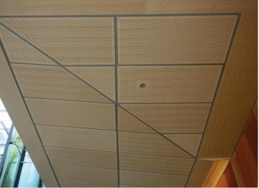
Flat Panel Series 2 (SS2) is a ceiling panel with reveal edge, sitting on Armstrong® Prelude® XL® grid to create 1" reveal between panels, or Suprafine® XL® grid for a 5/8" reveal. Panels are easily removable for accessibility above the ceiling.
