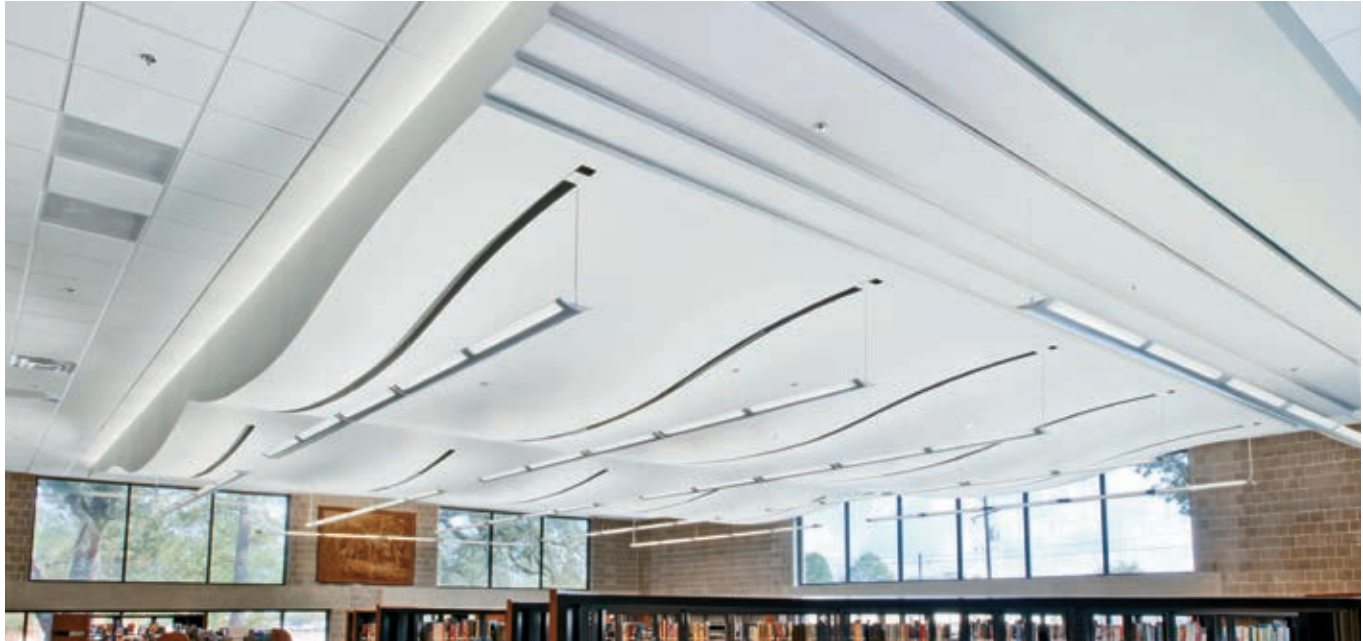
▲ Faceted Drywall Grid System for curved drywall ceilings
