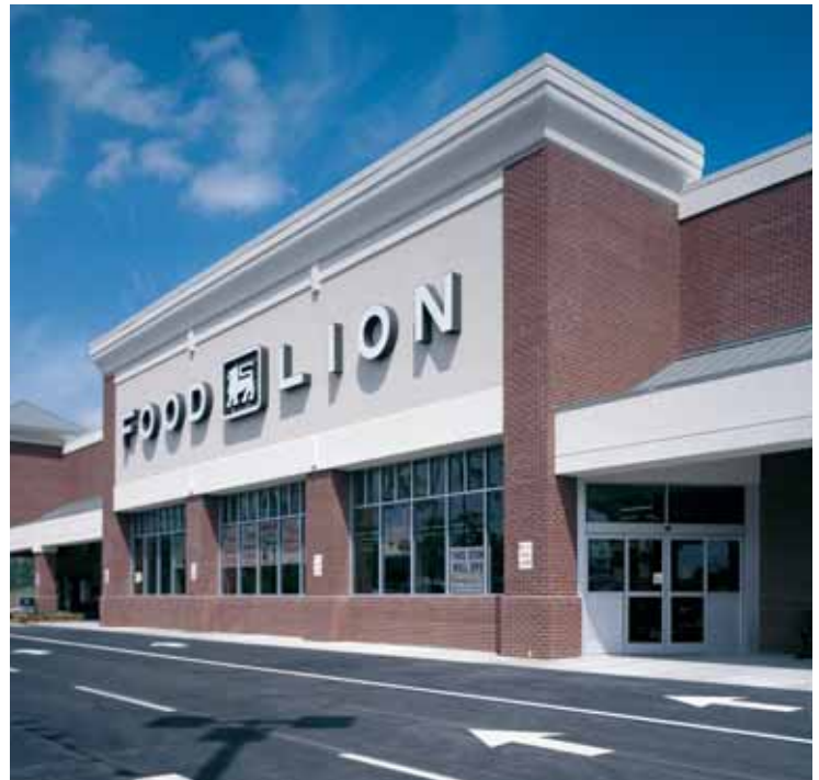
Ceiling recycling is now an integral part of every Food Lion renovation project. More than 100 stores, such as this one, could potentially be part of the program each year.
