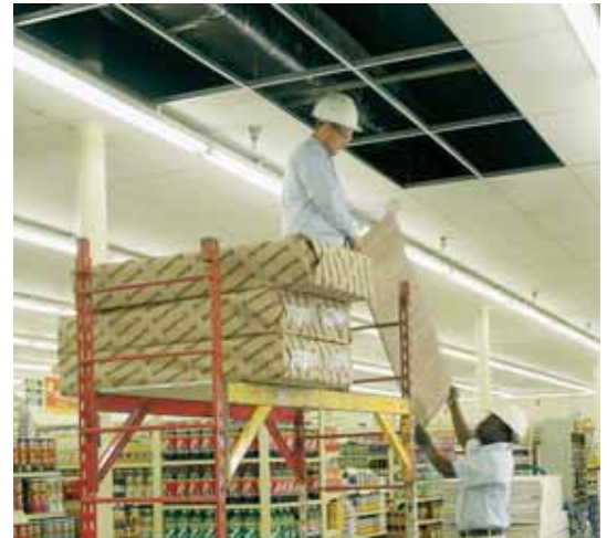
Ceiling tiles removed from a store will eventually be shipped to an Armstrong plant where they will be used as raw materials in the manufacture of new acoustical tiles.
