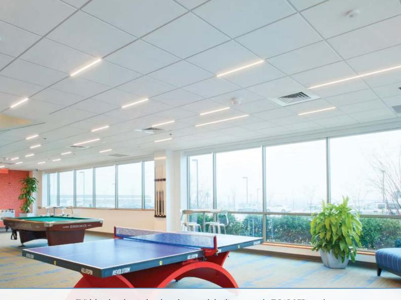
"With less than three inches above the suspended ceiling system, the T-BAR LED was the perfect fit due to its minimum plenum occupancy that directly integrates into the ceiling grid."
