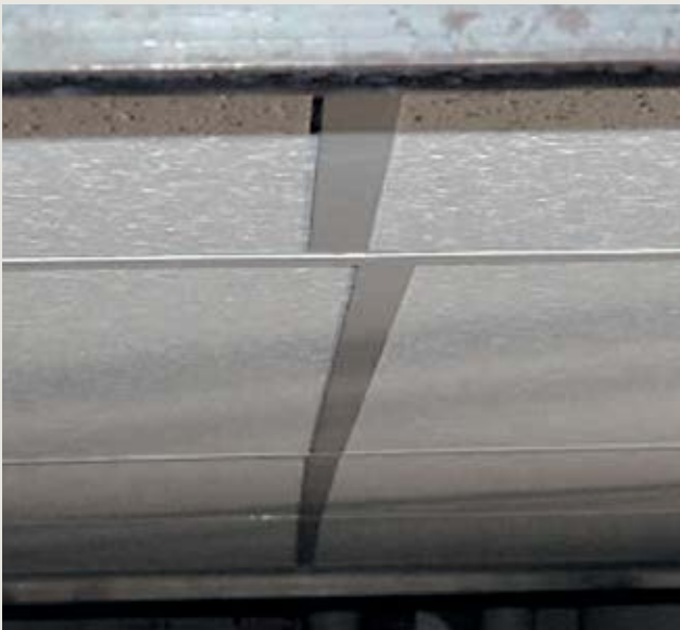
Damage at cross tee connections allows ceiling movement.
