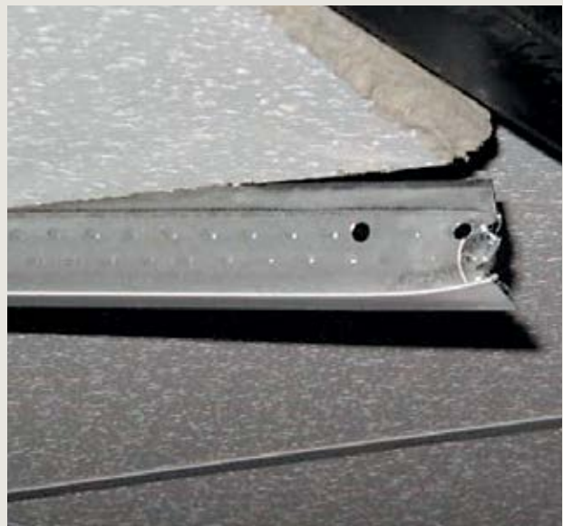
Unsupported cross tees allow panels to drop out.
