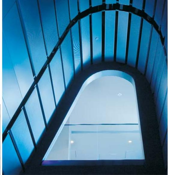
Custom Metal Walls unperforated and with Rd 1522 perforation in Custom RAL 7024 finish
