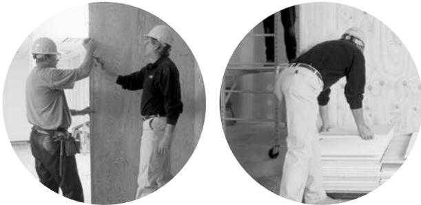
Many crews speed up the stacking by building a simple two-sided, free-standing frame. Note: Frame is not attached to pallet.
