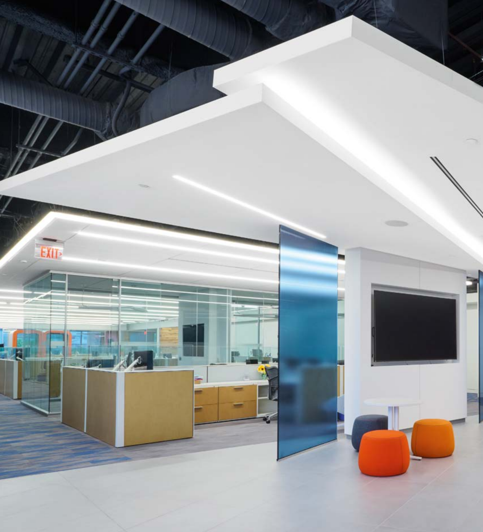
AcoustiBuilt Ceiling System; REGENXBIO Regional Office; Rockville, MD
