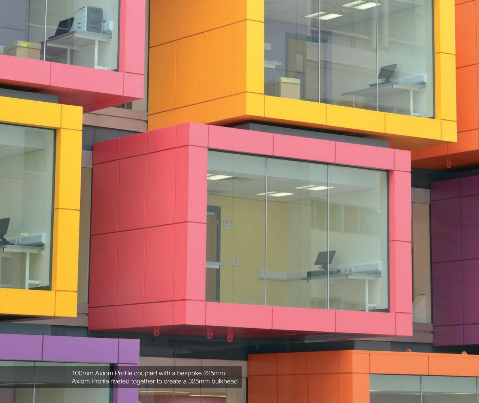
100mm Axiom Profile coupled with a bespoke 225mm Axiom Profile riveted together to create a 325mm bulkhead
