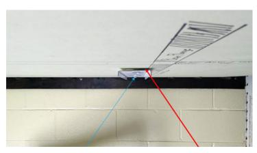
(Fig 3) Temporary Retaining Bracket installed Approx. 1/8" gap
