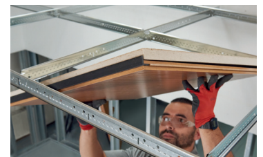
WoodWorks Channeled ceiling panel with Calla 2820 acoustic infill panel for Total Acoustics performance
