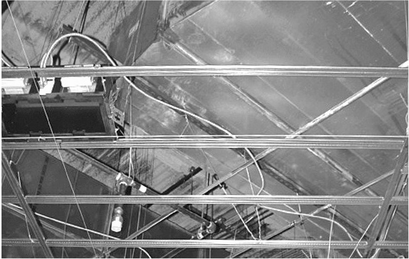
FrameAll grid system with the 6' cross tee, XL8965
