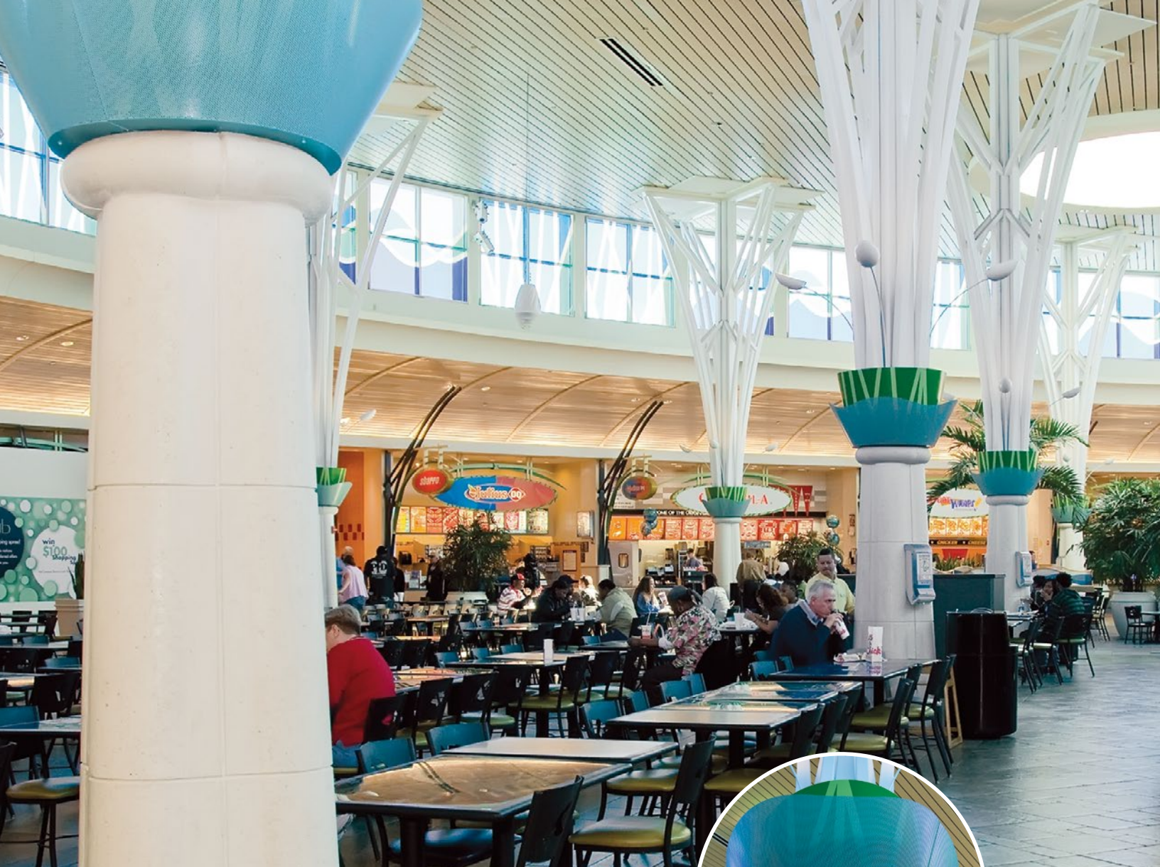
Interior Molded Stone column covers; Oglethorpe Mall, Savannah, GA; Thompson, Ventulett, Stainback & Associates
