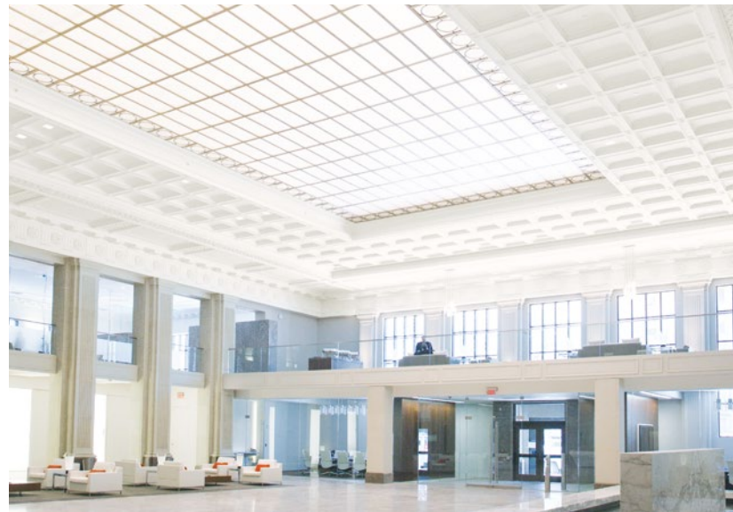
GRG coffers and cornices; The Rockwell Building, Cleveland, OH; Sandvick Architects and Vocon
