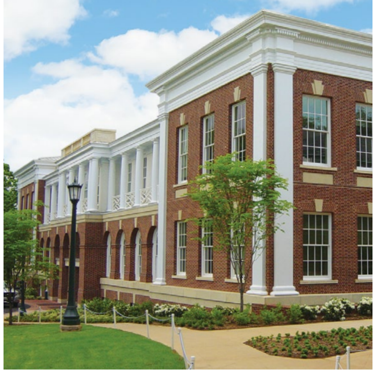
GFRC and GRG column covers, cornices, and various castings; UVA McIntire School of Commerce, Charlottesville, VA; Hartman-Cox Associates
