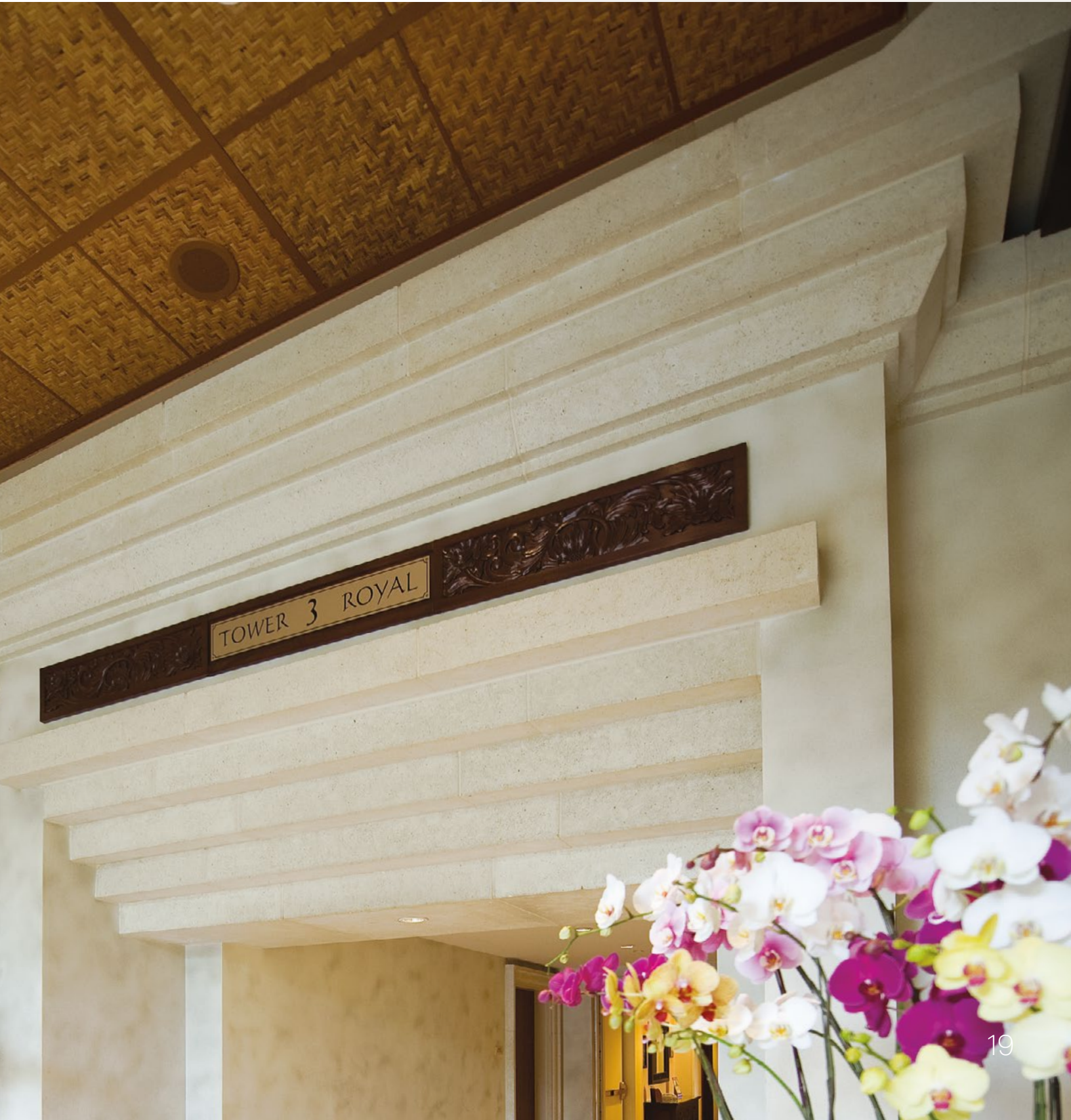
Interior Molded Stone cladding, headers, base, and door surround; Royal Pacific Resort, Orlando, FL; Fugleberg Koch Architects
