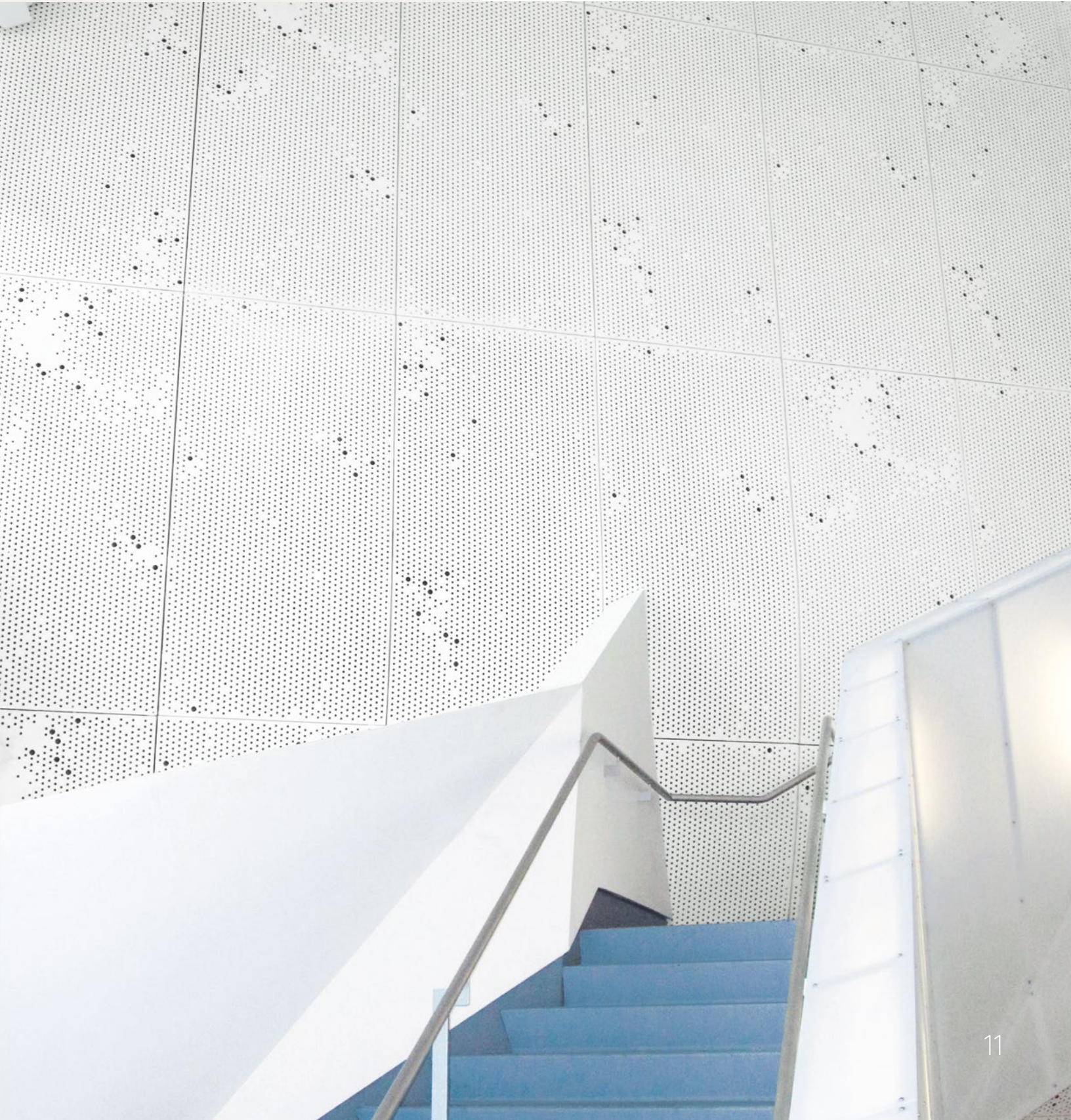
GRG randomly perforated wall panels The Cooper Union, New York, NY; Morphosis
