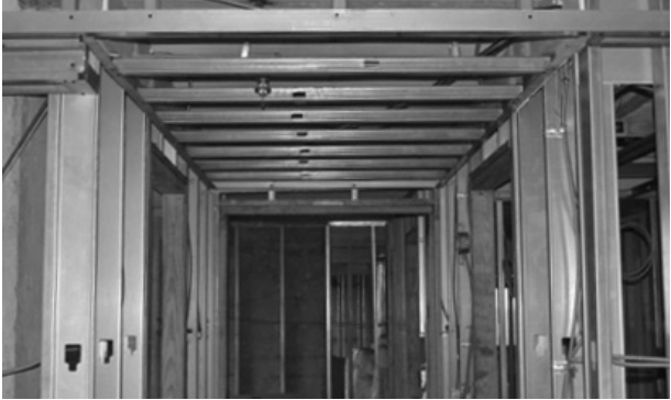
Corridor framing using traditional steel studs
