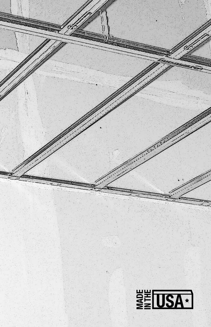
Flat Drywall Grid Installation
